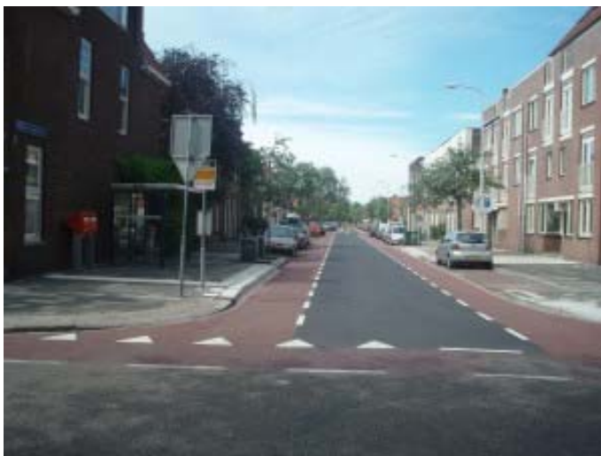
Typical Shared Bicycle Lanes- Pauwstraat in Delft
