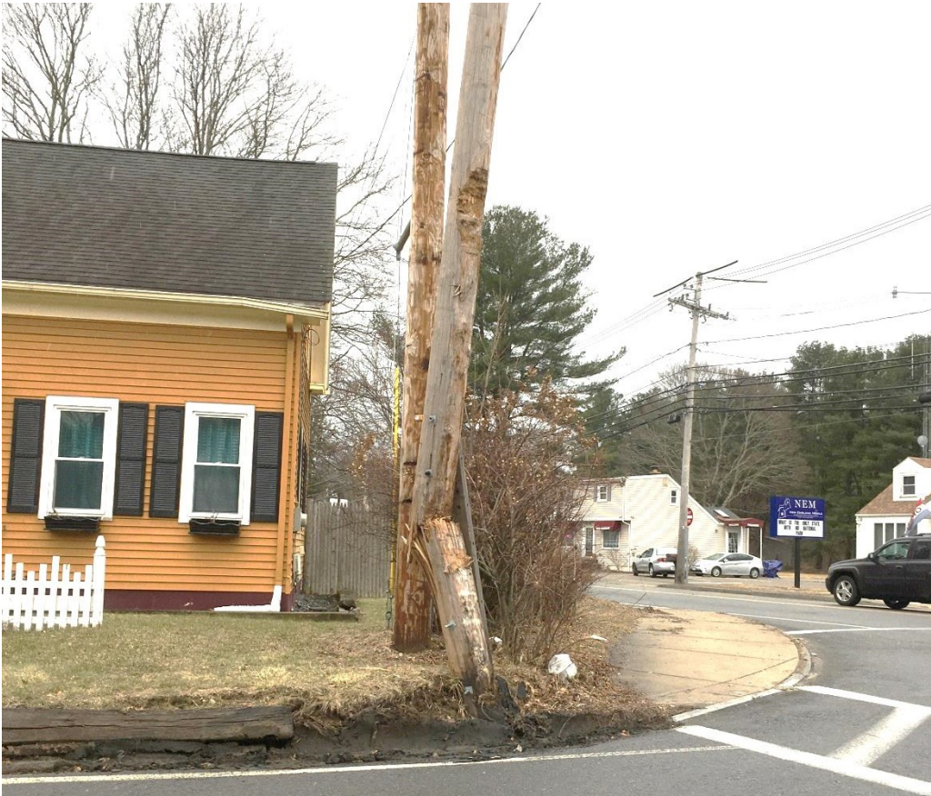
Figure 4 Telephone Pole in front of 3 Maple Street
