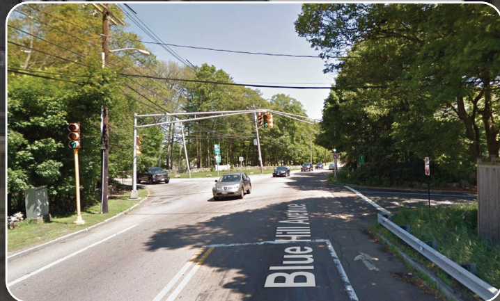
A picture of the existing roadway
