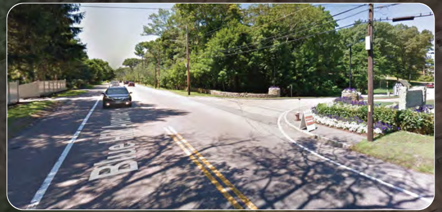
A picture of the existing roadway
