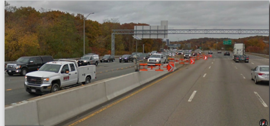
End of the southbound HOV zipper lane showing merge area (facing northbound)
