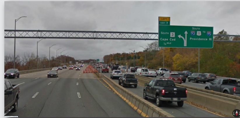
End of the southbound HOV zipper lane showing merge area (facing southbound)
