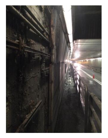
Delaminated Concrete & Corroded Ceiling Beams
