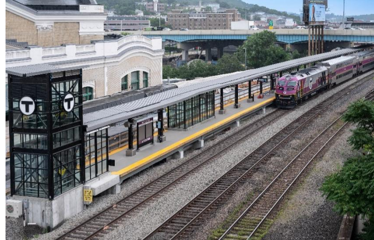
Commuter Rail train at new Worcester Station platforms
