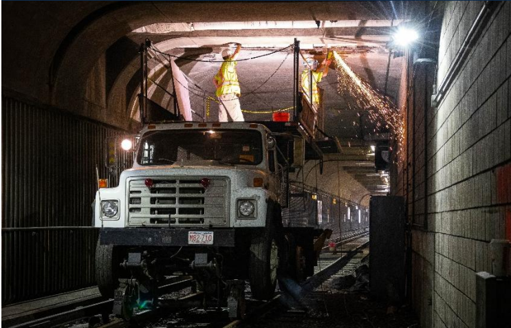
Orange Line tunnel repairs near Forest Hills Station
