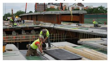
repair of structurally deficient bridges across the Commonwealth. It has used novel project development and construction techniques that deliver projects on an accelerated schedule. One such project that received national attention was "Fast 14," which replaced 14 bridges on Interstate 93 in one construction season by using prefabricated bridge deck panels.
