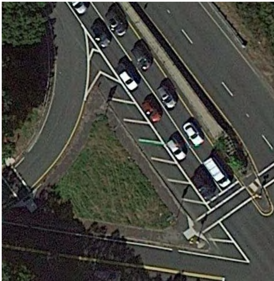
Figure 8 Existing Zebra-Striped Pavement on Route 2 Southbound
