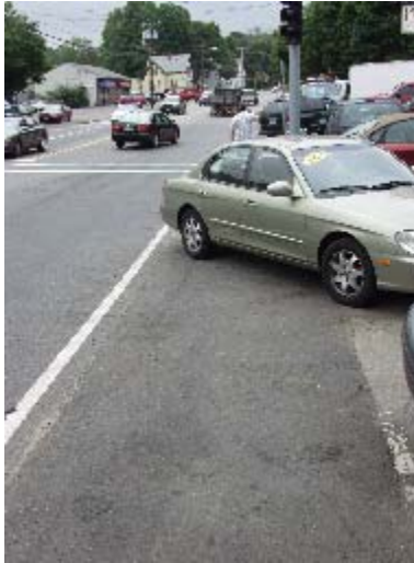
The sidewalk is not clearly separated from the roadway at the intersection of Pleasant and Water Streets
