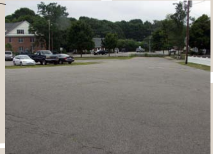
Large paved area
