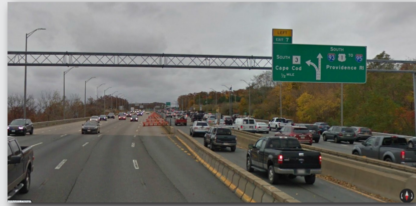
End of the southbound HOV zipper lane showing merge area (facing southbound)
