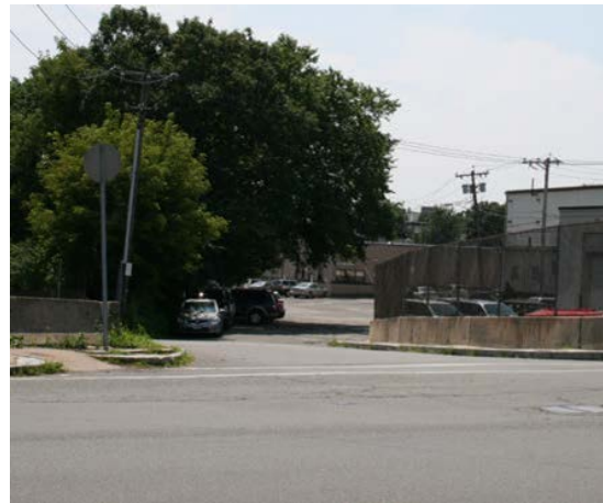
Winter Street: Missing pedestrian ramp at SW corner
