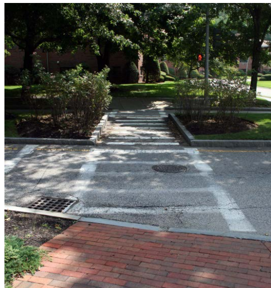
Grove Street: curb cut and ladder-style crosswalk in median
