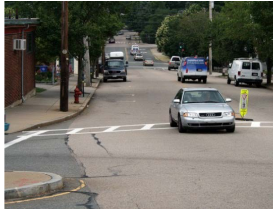
Lexington Street: Potential location for curb extensions
