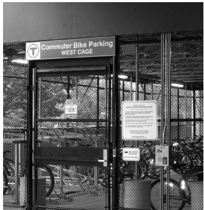
COMMUTER BIKE CAGE AT MBTA STATION
